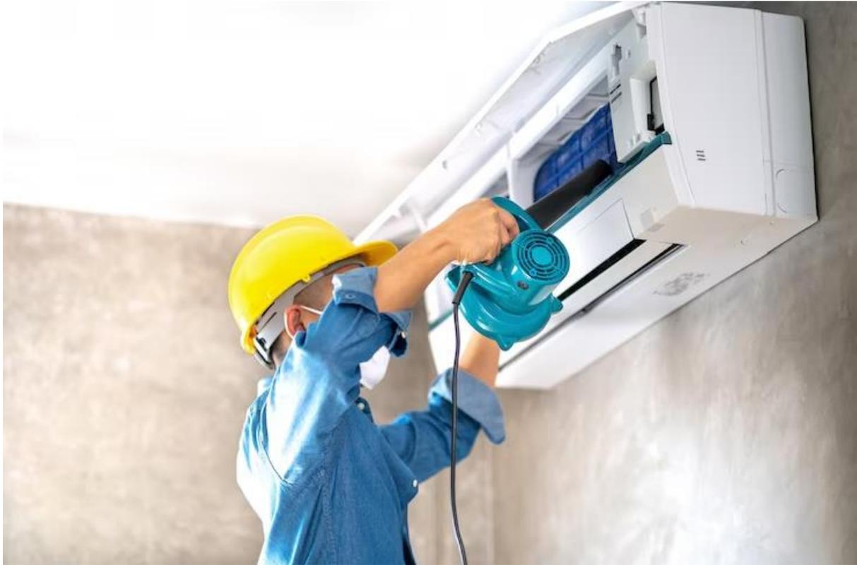
1. **Compressor switching off regularly** – This becomes a problem for most people who live in cities and pollution is rampant. When dust and dirt accumulate and choke the AC filter, the AC starts to work harder for air intake and this results in increasing pressure on the compressor. You can try to open the AC from time to time and clean the dust accumulation but it would be better to call on professional split AC repair services in Bhubaneswar and let them take care of it.
